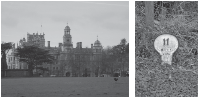
Fig. 1 Two examples of listed buildings in Nottinghamshire: The large 19th century country house Thoresby Hall and the late 18th century cast-iron mile post at the Grantham Canal near Kinoulton.
